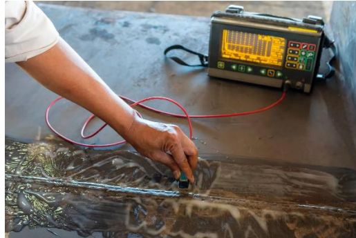
Fig. 1.3.25: Ultrasonic testing of weld [1.3.34]
